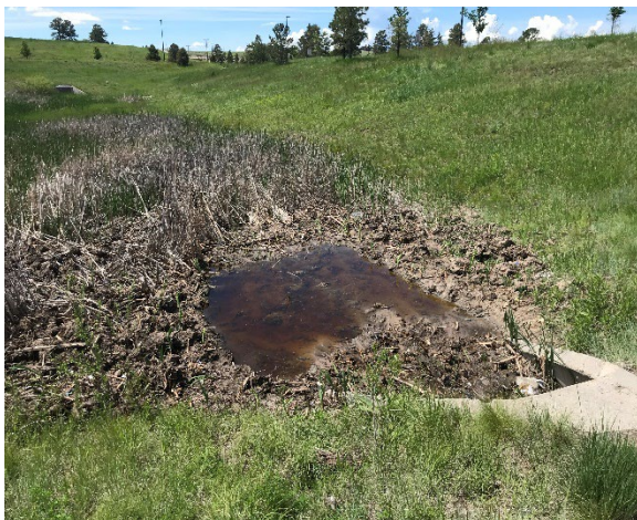
The cattails were removed. This method is not recommended, cutting flush with the ground is recommended - South Pond, north inlet.
