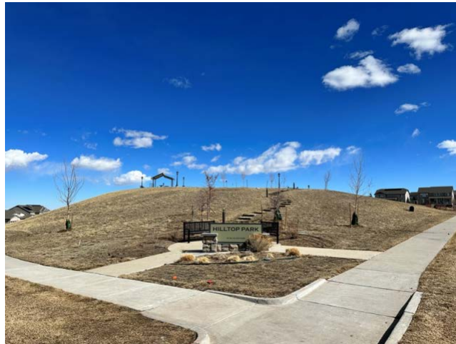
This is for the replacement of the stone and metal monument sign at the Hilltop Park.
